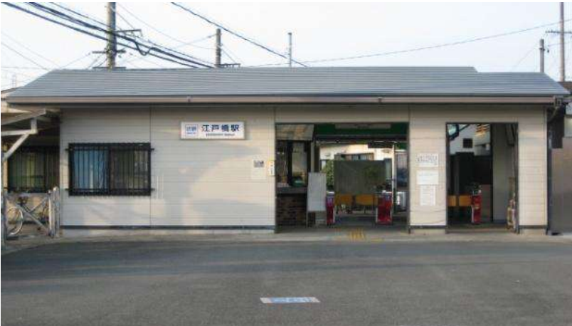
Existing Edobashi station entrance
